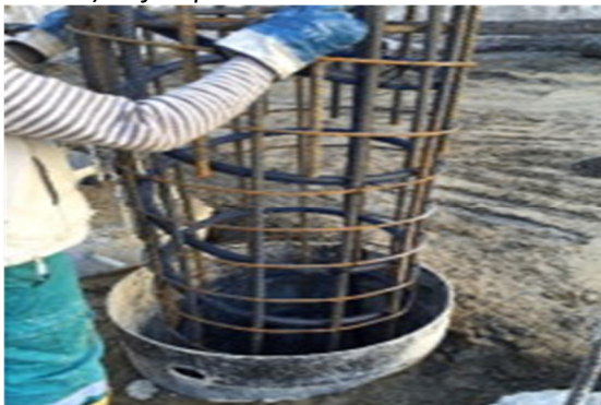
Energetski pilot ( \approx 1 - 3 \text{ kW} na pilot) https://ars.els-cdn.com
